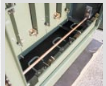
Deadfront Fuses Utilize Elbow Connectors for 200-Amp Switching
