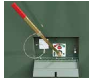
Switch-Handle Operation - handle unfolds and clip slides over joint to fix handle in extended position
