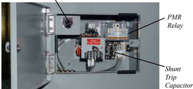
Figure 11. Shunt-Trip Switch Control Components.
