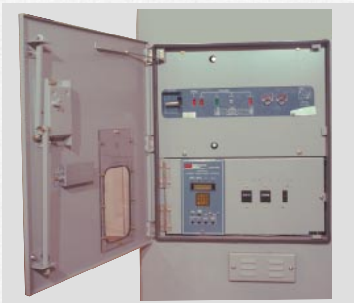
Low Voltage Control Compartments Contain Switch Operators and Microprocessor-Based Control for Automatic Source Transfer
