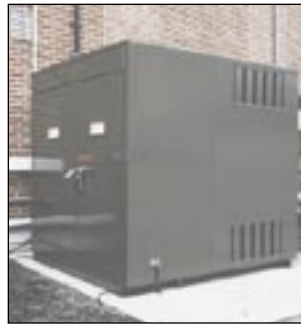
Padmounted Transformer
